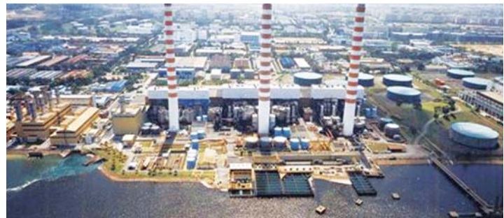
Aerial view of Senoko Power Station
