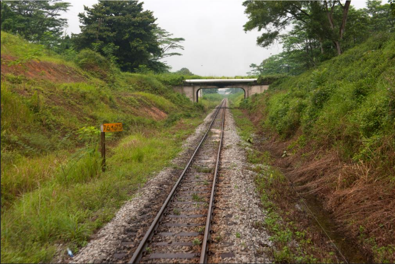
Concrete Bridge across former KTM railway line (Kranji section) in 2011 (Source: URA)
