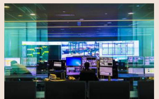
Remotely supervise up to 5 cranes in Automated Crane Operations Centre and handle exceptions
