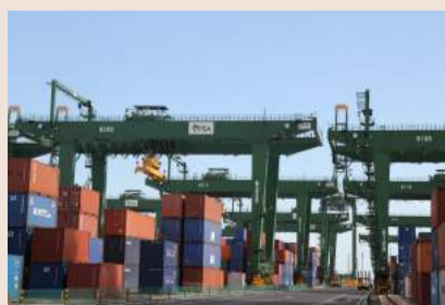
Remote yard crane to increase productivity
